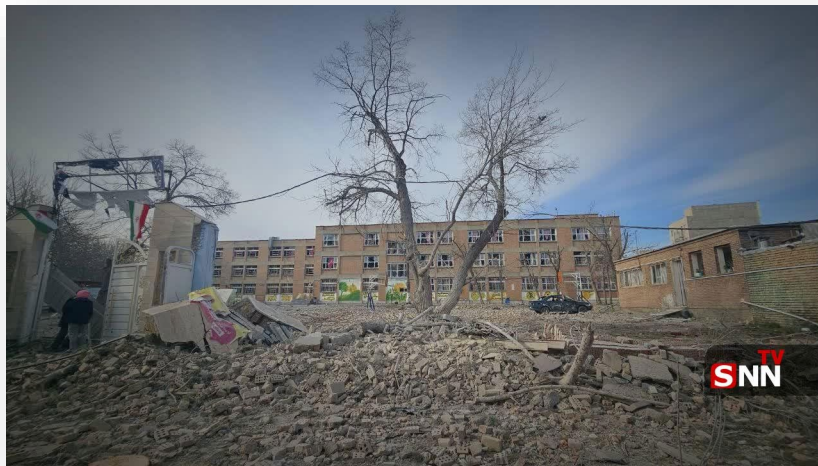
A snapshot of the rubble of Esmat girls' school in Urmia, in north-western Iran, which was severely damaged by the US and Israeli regime's air raids.
